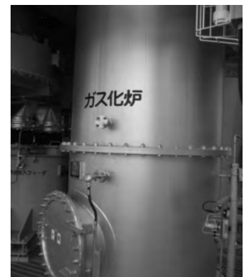
Fig. 3 Gasification furnace
