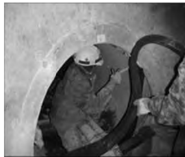
Photo 4: Installation of seismic-resistant materials
