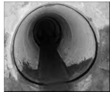
Photo 5: Completion of seismic retrofitting
